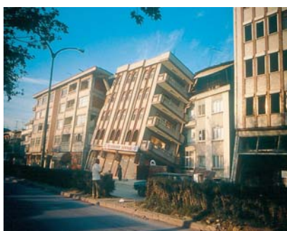
Fig. 2 This inclined building sank unevenly and leans against a neighbouring building
